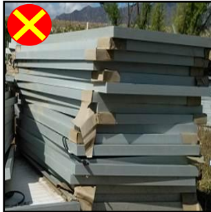
图 8.4-3 组件拆箱后堆放不整齐 Modules are not stacked neatly after being unpacked
