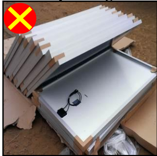
图 8.4-1 拆箱错误组件倾倒 Wrong way of unpacking causes modules to fall over
